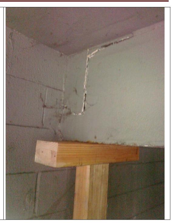
Close up of initial Dryrot on Glulam. Do to potential safety risk immediatel y purchased additional post and shored up glulam 6' back before opening up additional stucco to assess full damage of dry-rot.
