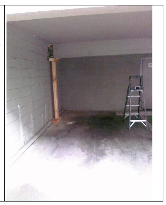
Initial view of glulam after temporary shoring for safety prior to removal of stucco to assess damage.
