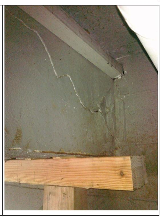
Outside wall causing the water to get inside Close up of ground/ electrical penetration into block wall.
