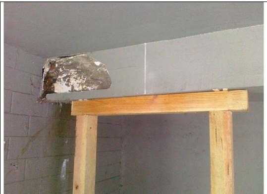
View of dryrot damage not including the glulam part on the block wall its self.
